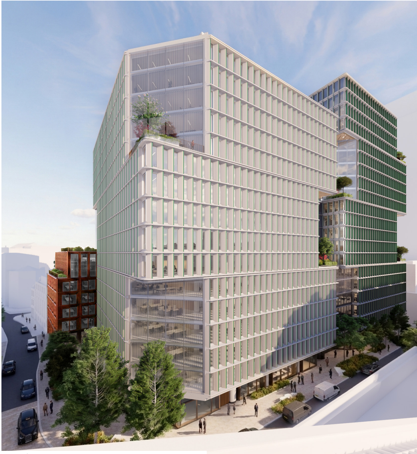
View of the South West Corner
