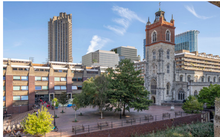
Southern Approach from London Wall The building's orthogonal massing and chamfered corners references the Barbican's own mix of angled and rectilinear geometry. Visible from Wallside Highwalk, the building offers a sympathetic wayfinding to assist in navigation through Barbican.
