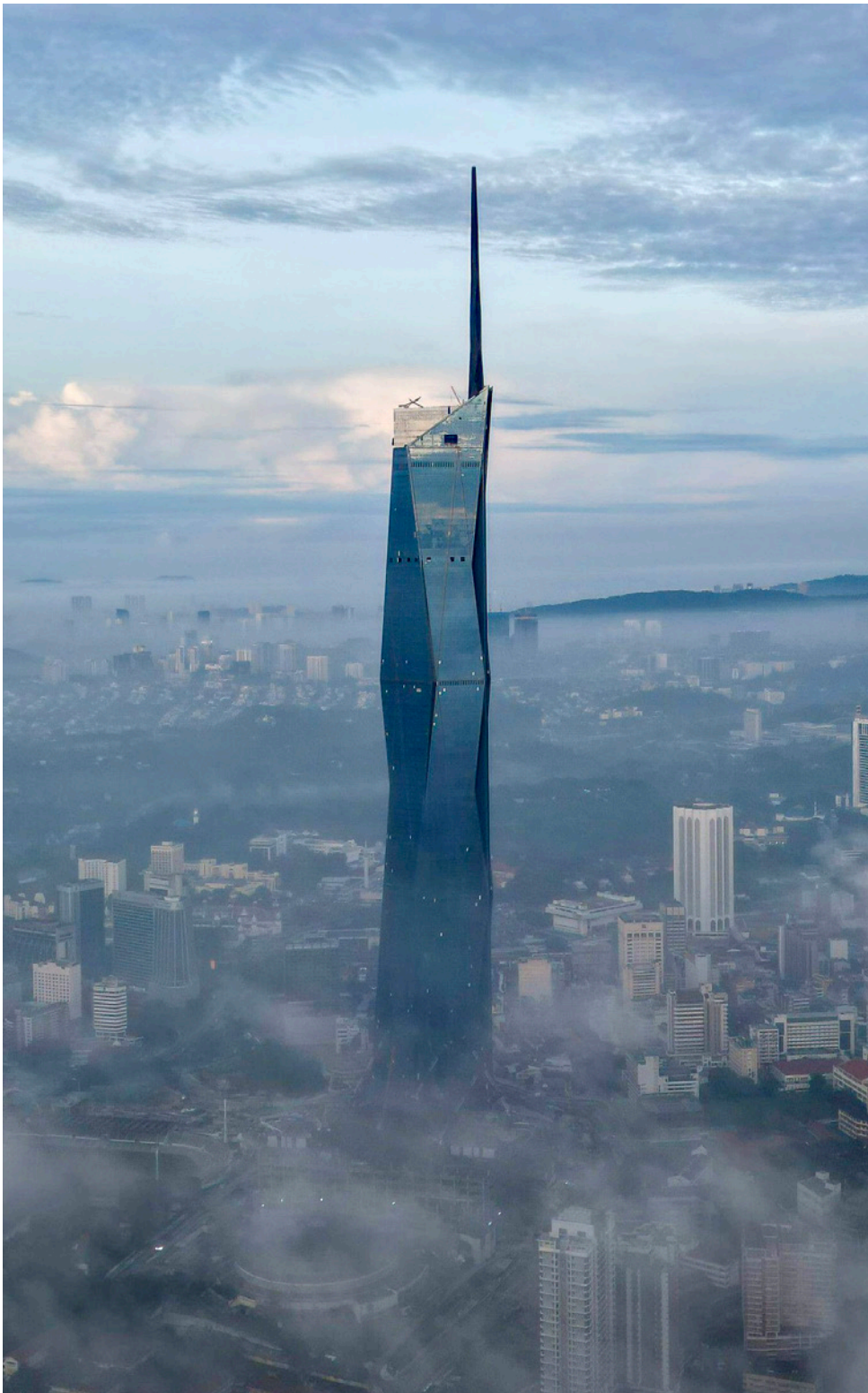
Merdeka Tower, Kuala Lumpur
