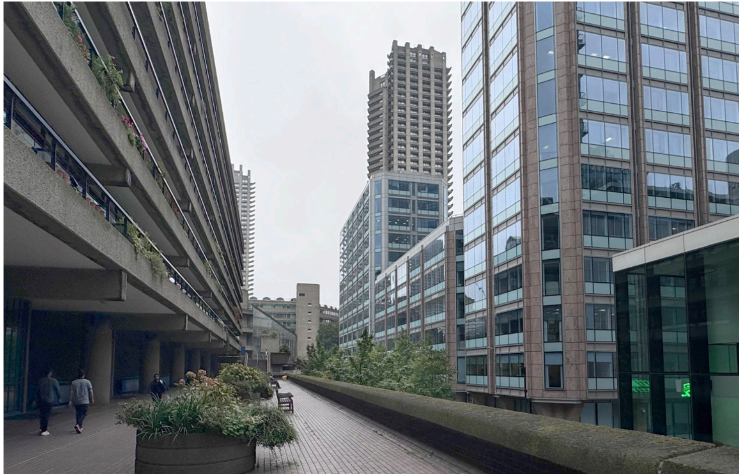
View of Existing Building From Speed House Highwalk
