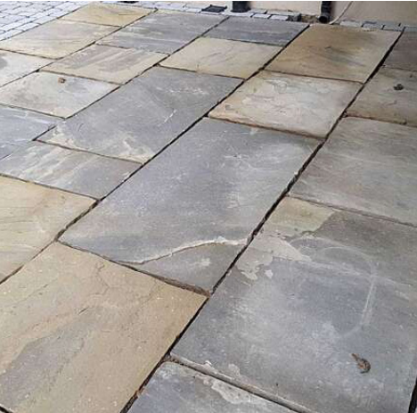
Natural stone pavers on sand bed
