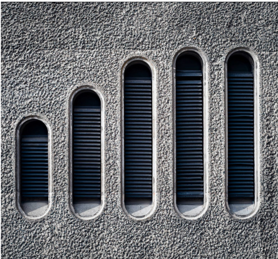
Crafted Vents Within the Bush Hammered Concrete Walls
