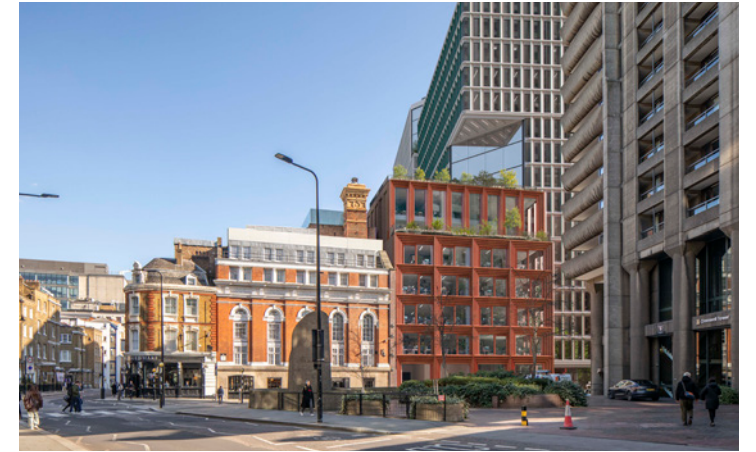
At the intersection of Whitecross Street, Silk Street, Beech Street and Chiswell Street, the set back of the building's massing is visible, revealing a civic plaza and the entrance to the Barbican Centre. The colour and reflections of the Brewery Annex's glazed terracotta frontage announces its cultural purpose and acts as marker.
