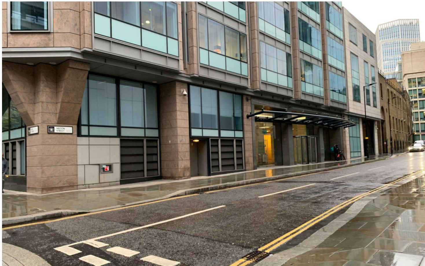
View of Inactive Ground Level Frontages of Existing Building Along Milton Street
