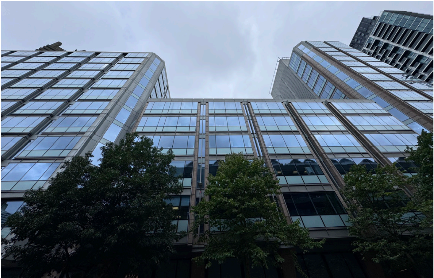
View Looking Up at Existing Building From Silk Street
